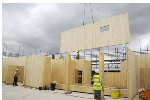
Photo 2: On site building assembly with CLT panels
